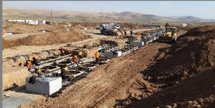
KRG MoE, Ministry of Electricity, Bazian, Süleymaniye/ IRAQ 132/11 kV Bazian Switching SS The Construction of High-Voltage Switchgear
